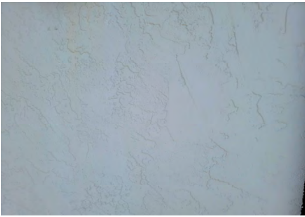
25 Exterior Paint Overview
