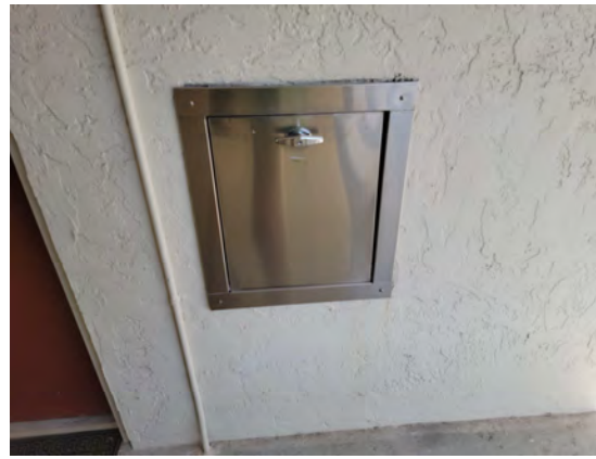
42 Trash Chute Exterior
