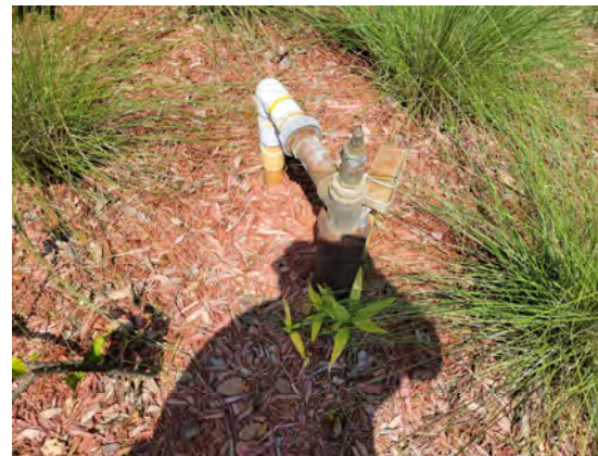
78 Main Water Shut Off
