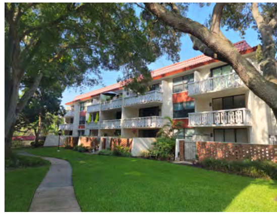
2 Right Side of Building
