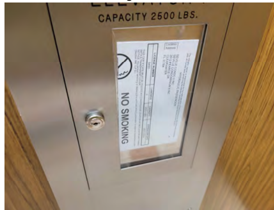
38 Elevator Cab Permit
