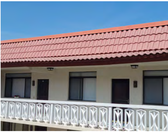
9 Mansard Roof Overview
