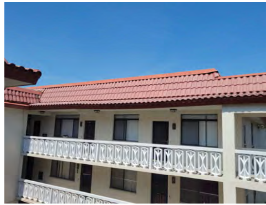
10 Mansard Roof Overview
