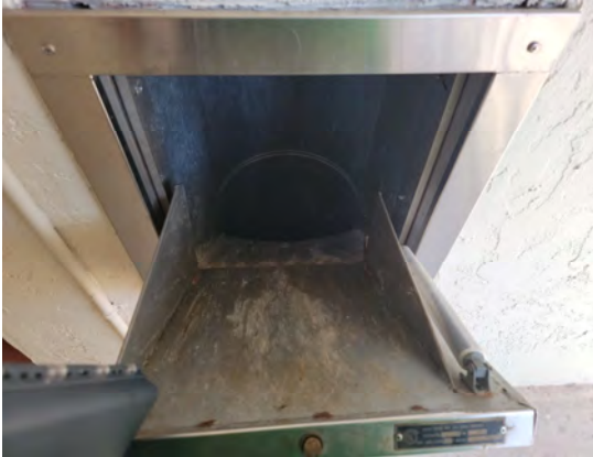
43 Trash Chute Interior
