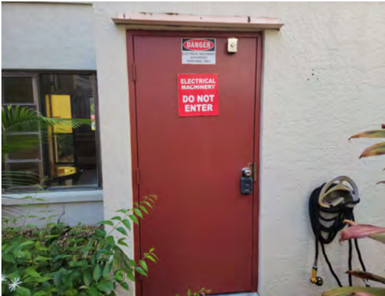
67 Mechanical Room Door
