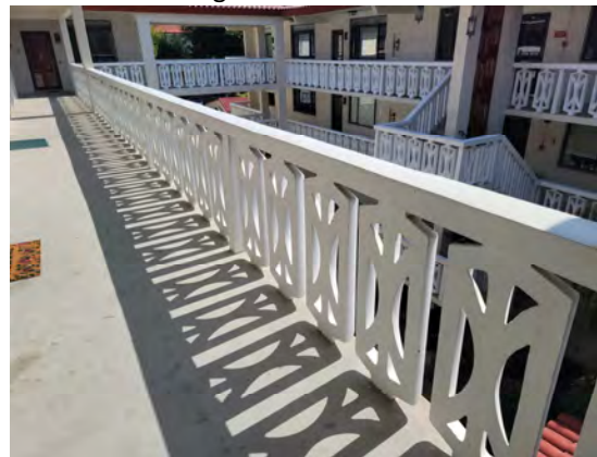
46 Walkway Railing Overview
