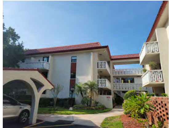
4 Left Side of Building
